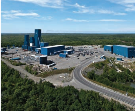
Aerial view of Glencore's Nickel Rim South mine near Sudbury. CREDIT: GLENCORE
