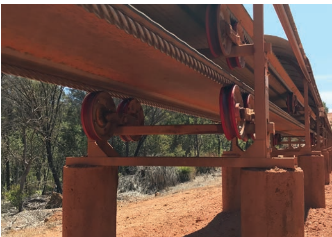
Cable belt (Boddington). CREDIT: CONVEYOR DYNAMICS
