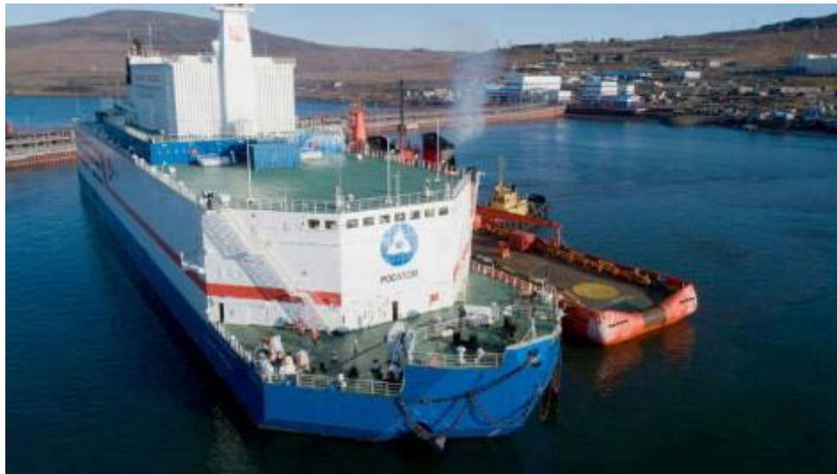
Figure 3 Akademik Lomonosov floating nuclear power plant
